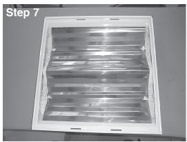
7. Remove protective film from reflector insert lamps.
