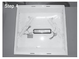
4. Properly connect ballast and lamp holders into new brackets.
