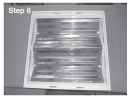
6. Insert reflector into the outer tabs on new bracket. For ease of installation squeeze the reflector tab into the middle and snap into tab.
